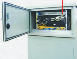
Easy mounting specific designed outdoor enclosure is put over existing street cabinet
